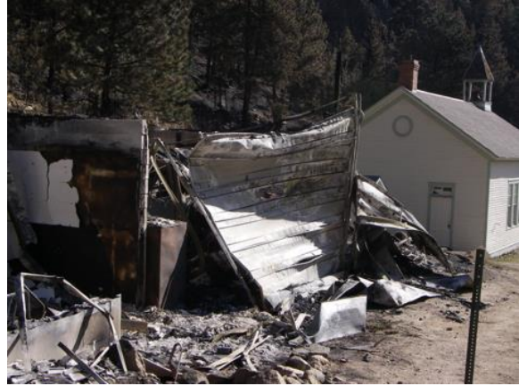
Figure 3. The burned-down fire station by the Salina Schoolhouse.
