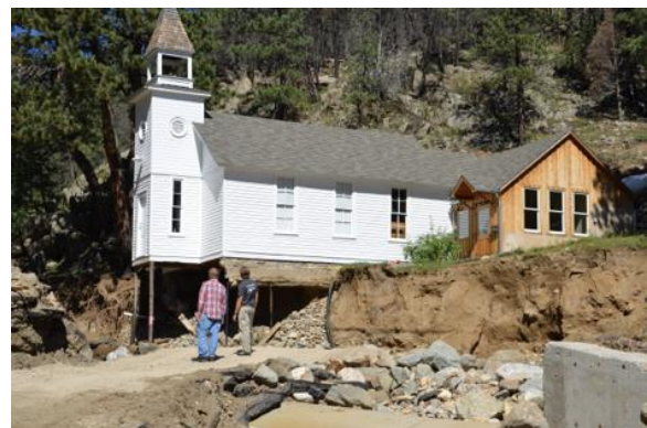
Figure 5. The Little Church in the Pines which was undercut by the flooding.
